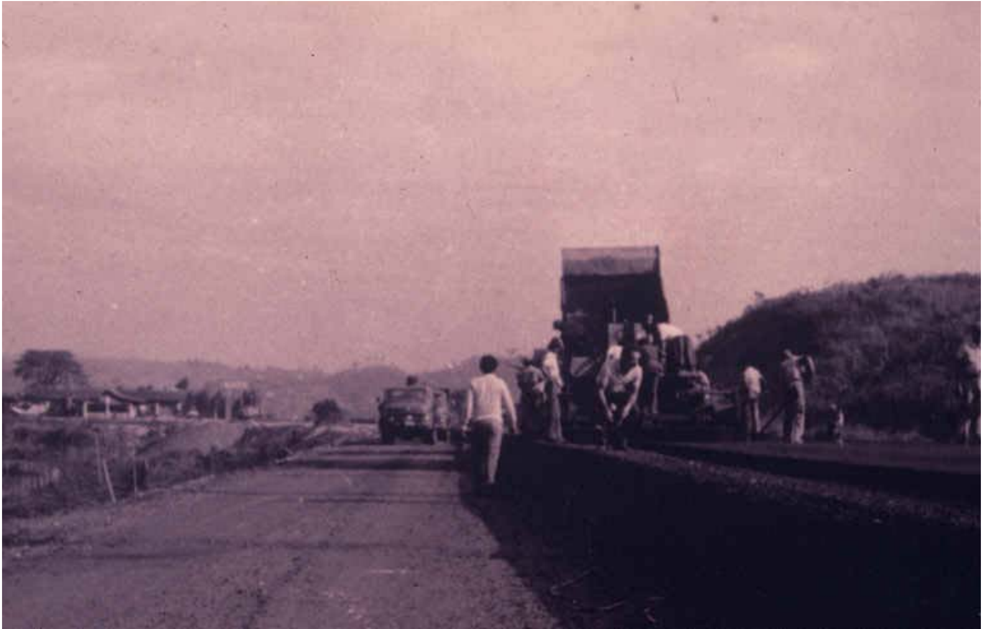
A bituminous overlay on BR-040 in Brazil
